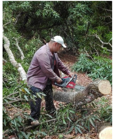
Clearing the new building site
