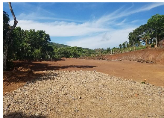
Newly extended driveway and pad for the building
